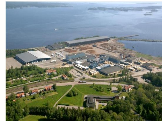
Pyrocell Setra, Gävle Sweden
